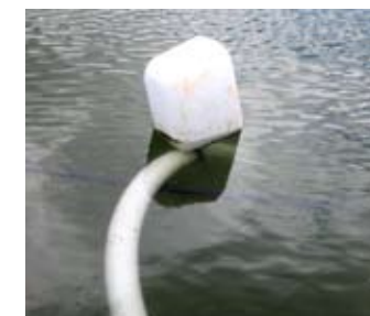
Flloating pipe to prevent mud entering the system
