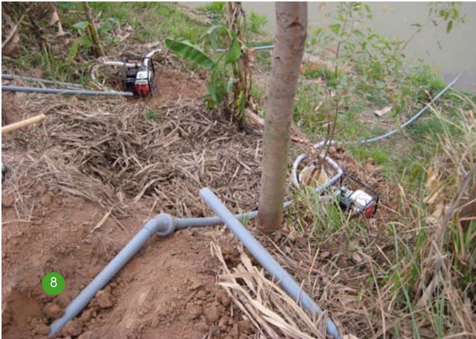
Place pump as close as possible to river
