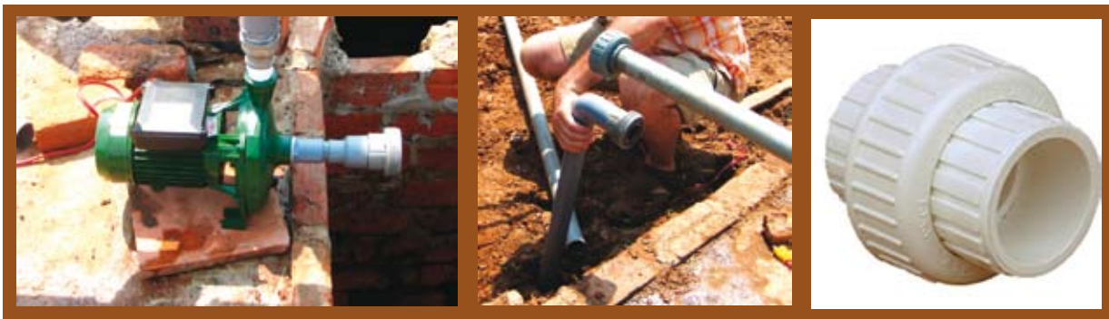
Screwing pipe union piece for mobile pumps
