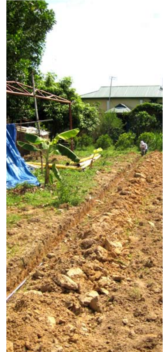
Trenches for the main-line
