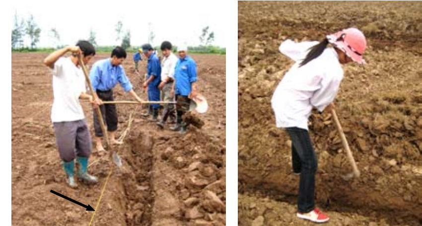
Excavating the trenches for the underground pipe network
