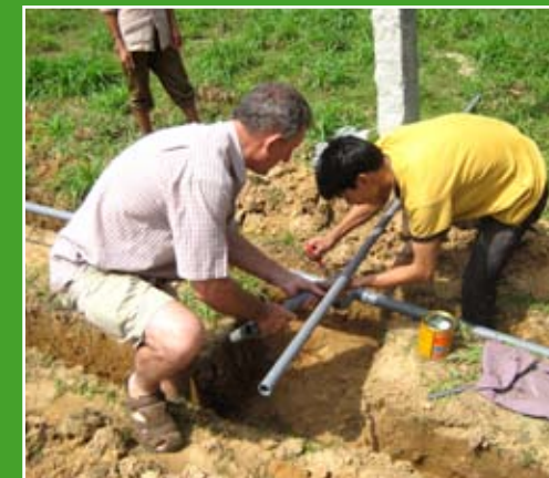
Cut main-line and connect with the sub-line
